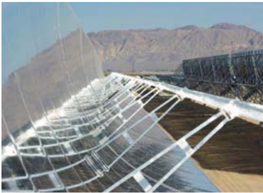
The SkyTrough is made from one single sheet in the transverse direction. That avoids alignment errors.
