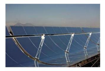
18 months of operation of a 1 MWth demonstration loop in SEGS II A 8m width and 150m length will be the optimum trough by 2014
