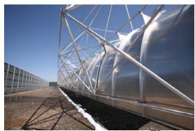
Figure 2 – back side view of the SkyTrough<sup>TM</sup> space frame
