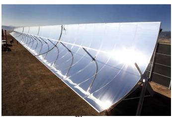
Figure 1 – SkyTrough<sup>TM</sup> SCA, Tracking the Sun
