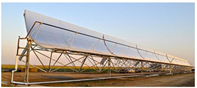
SkyFuel's high performance, low cost SkyTrough® parabolic trough solar collector, supplying heat to WaterFX desalination system .
