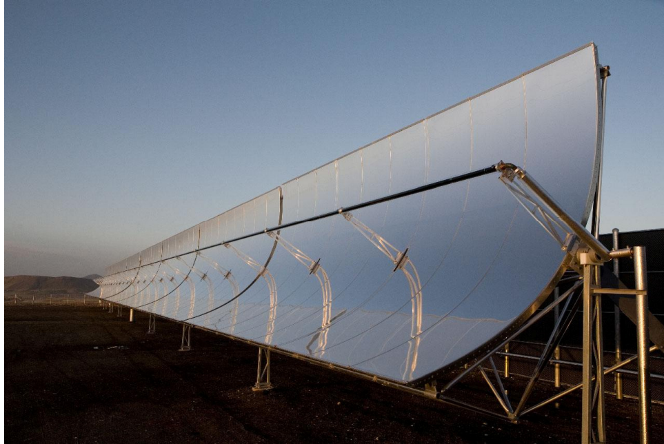
Figure 1. The SkyTrough Solar Collector Assembly (SCA), comprised of eight modules actuated by a central drive.
